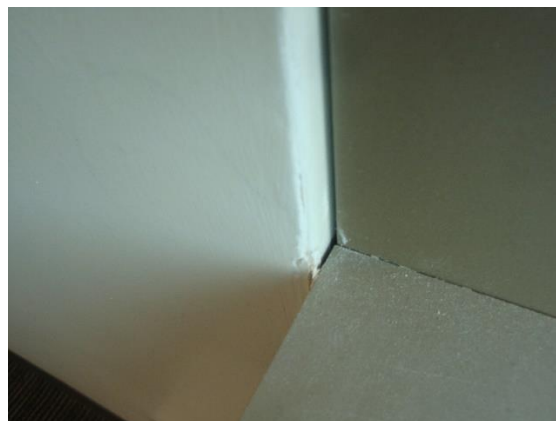
Figure 66: The gap in the same wall shown in figure 65, where the wall meets the window
